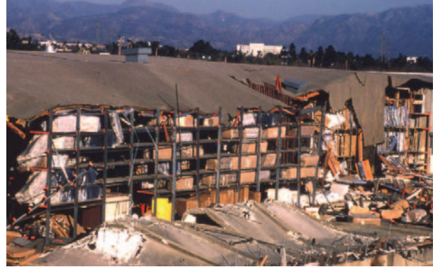
Collapsed Tilt-Ups.
