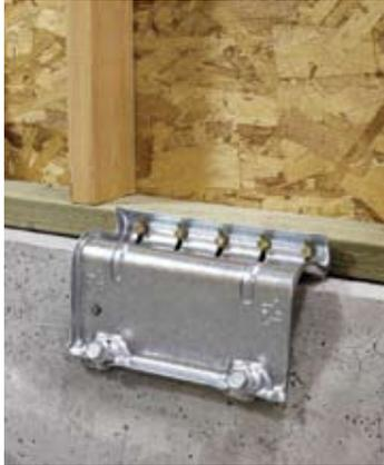
**UFP Installation, Anchoring the Mud sill to the Foundation**
